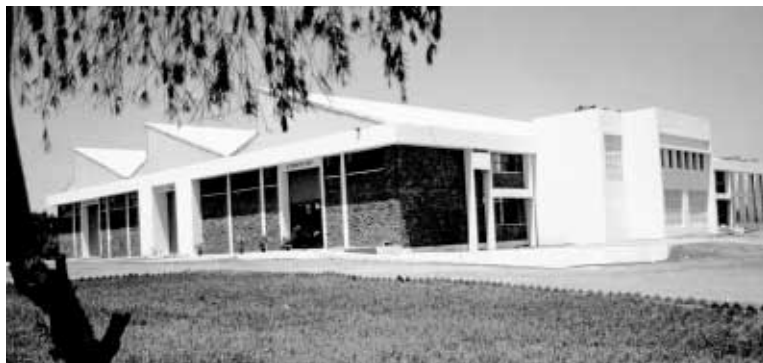
The Ahmednagar factory - manufacturing DC Motors
