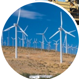
Wind Mill Generator
